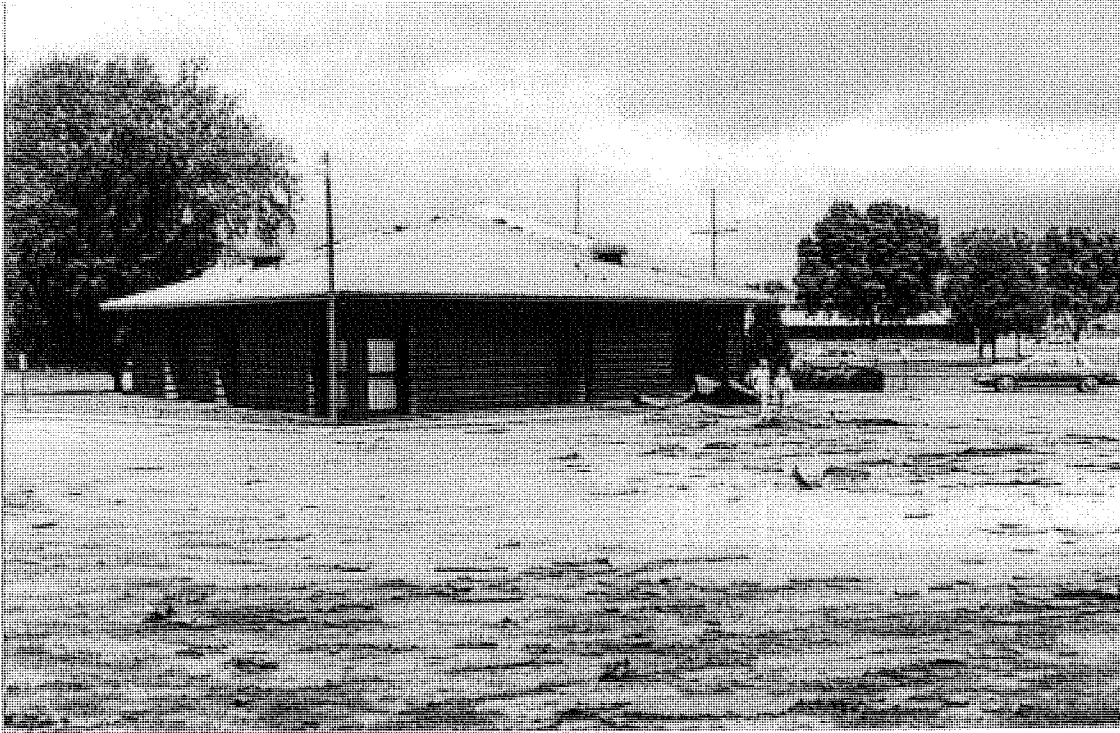
Straight-line wind damage in the June, 1990
