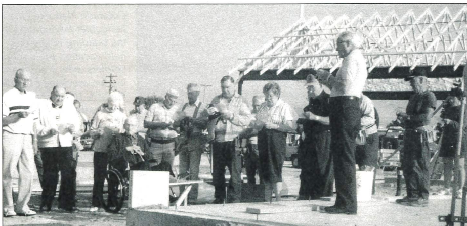
Leonard Buelow, pastor of Christ the King, held a short worship service for the cornerstone laying of the new church. This is the first church building for Christ the King. Previously the congregation worshiped in a grade school.
