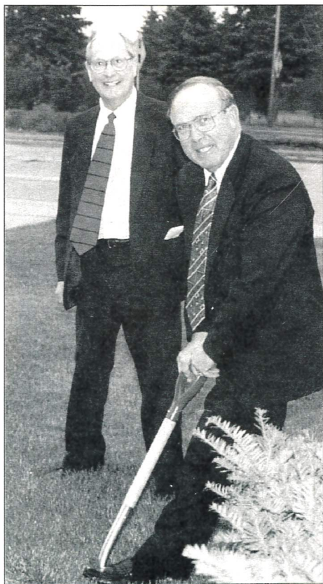
President Karl R. Gurgel (right) and Clair Ochs, Board of Trustees administrator, break ground for the WELS administration building expansion. The expansion will allow for handicapped accessibility.
