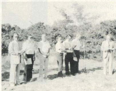
Groundbreaking at Gethsemane
