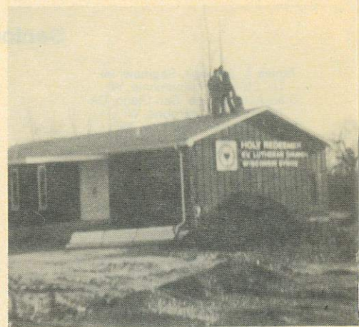
Members erecting the steeple
