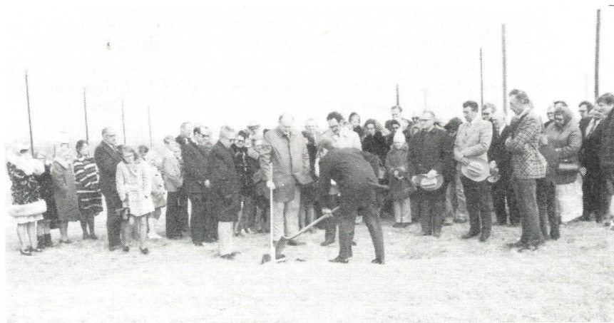
Groundbreaking at Valentine. Pastor R. Kugler wielding the shovel.
