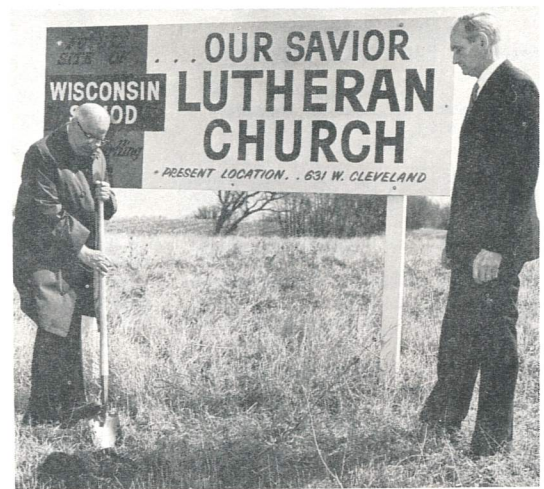
Groundbreaking at Freeport, Illinois — Pastor F. E. Bartling (left) and Mr. Walter Schult, chairman of Our Savior Lutheran Church.
