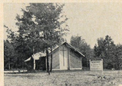
REDEEMER EV. LUTHERAN CHURCH of Tomahawk, Wisconsin, presents this exterior appearance.
