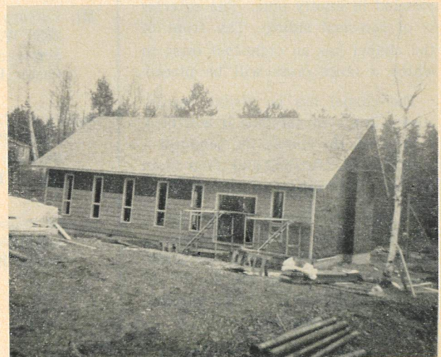
November 16. Redeemer Lutheran, Tomahawk, soon will have a home.
