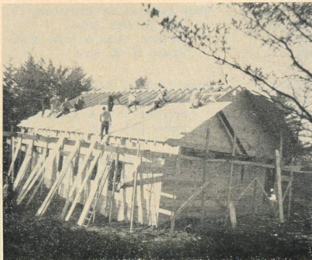
A week later, October 27. The building is almost under roof.
