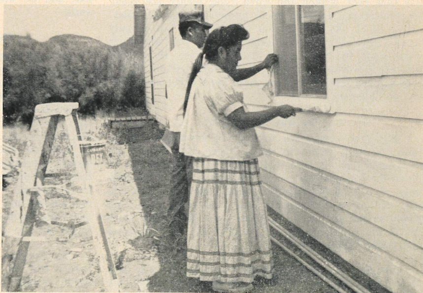
PAINTING THE NEW ADDITION are Terry and Andre Cosey
