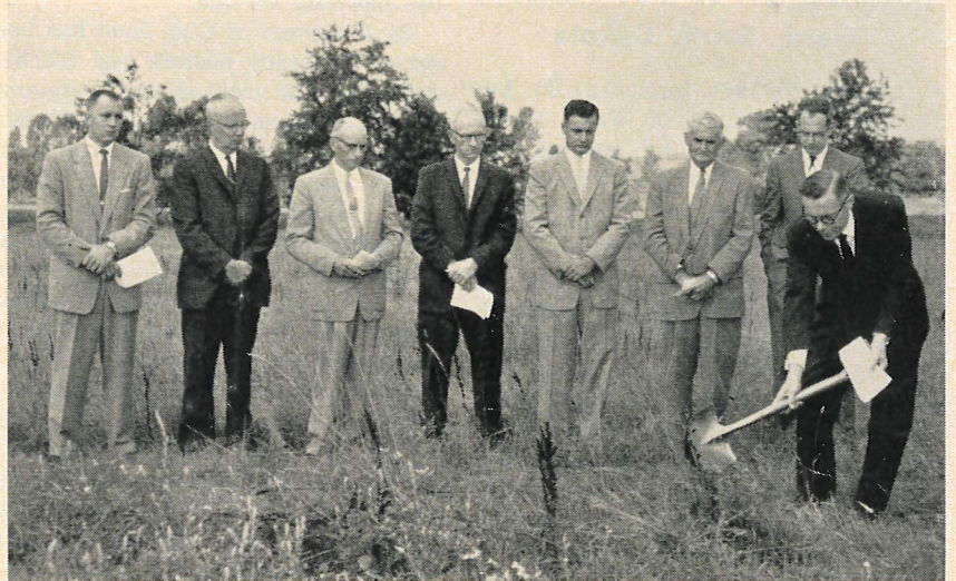
Groundbreaking for new St. John's School, Burlington, Wisconsin
