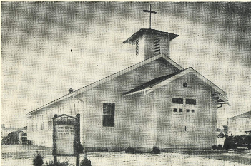
The Temporary Chapel Without Basement
