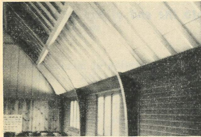
LAMINATED TRUSS CONSTRUCTION BEAUTIFIES CHAPEL
