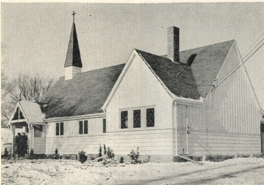
ENTRANCE AND SACRISTY SIDE OF CHAPEL
