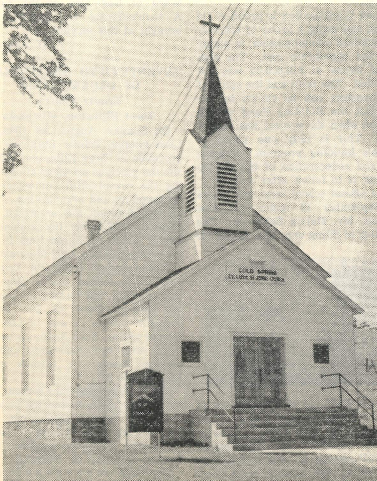
St. John's Ev. Lutheran Church
