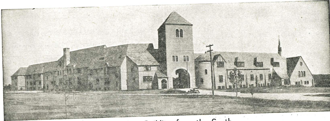
The Main Building from the South
