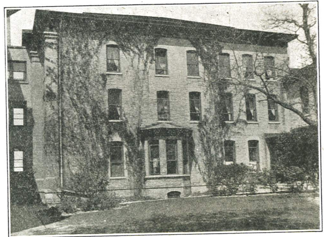
The Old Dormitory, which this year is exactly 50 years old. The passageway at the left leads to the new dormitory, which was erected in 1905
