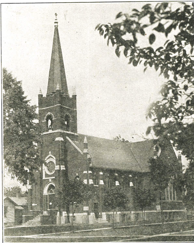
Trinity Evangelical Lutheran Church at Jenera, Ohio
