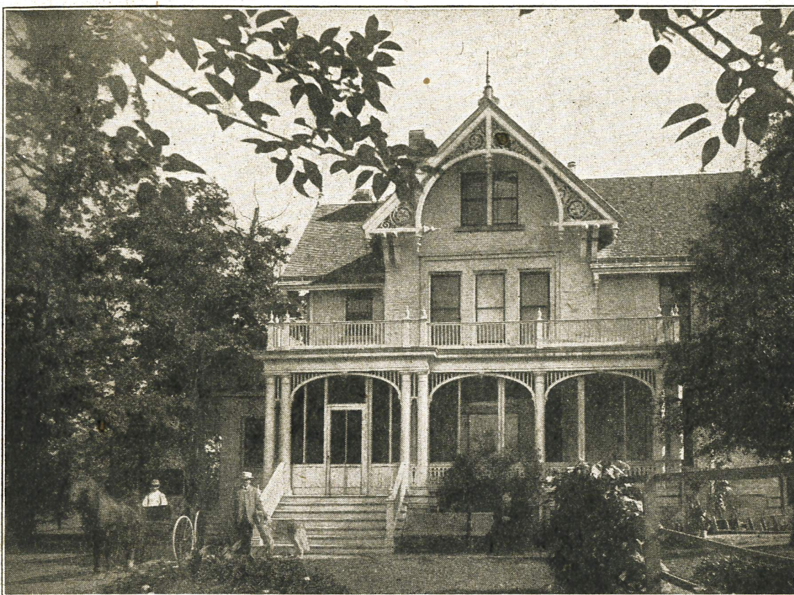
Residence On Our New Seminary Site—Bues Farm
