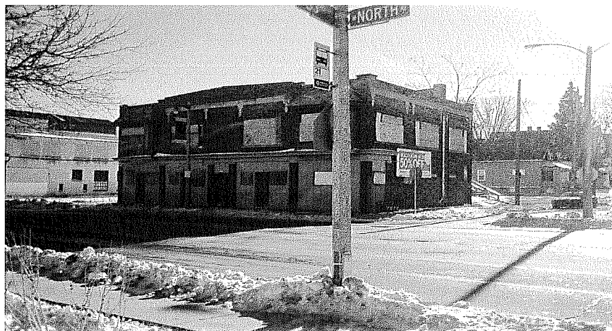
Picture #4 is a picture of a condemned building – found directly across the street from the newly constructed Todd Wehr Metcalfe Community Center. Sights like these are becoming harder to find as the neighborhood rebuilds.
