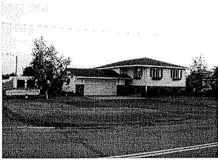
The present parsonage, built in 1989, located on the church property.
