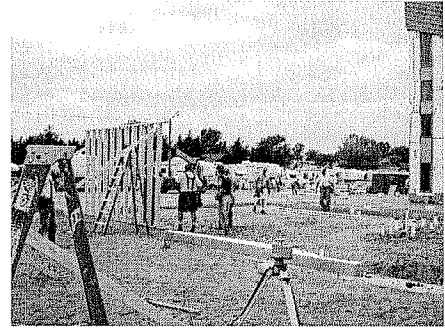
Builders for Christ at work, summer, 2006.
