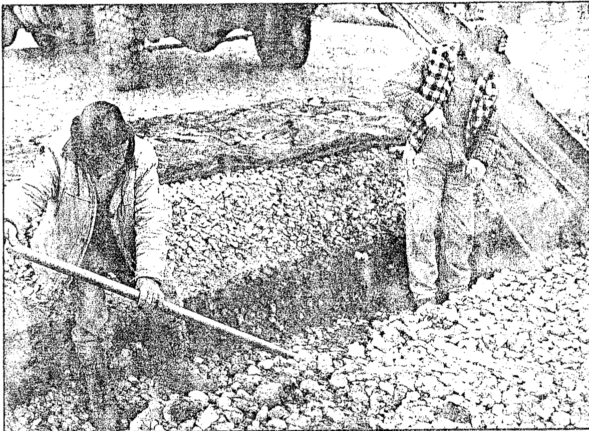
Jerry Peters, left, and Craig Jones of Concrete Masonry, spread concrete for footings of the Morning Star School being built on Highland Road in Jackson. (Staff photo: Chad Hug)
