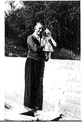
Wilfred Davis with child on the blocks of the foundation.
