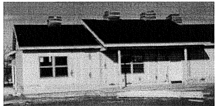
Parsonage under construction
