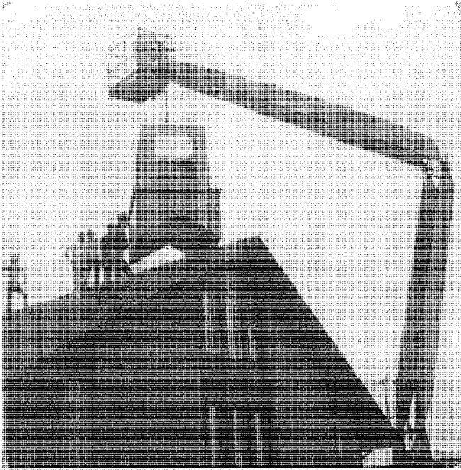
Steeple installed by OSLC members in summer 1973
